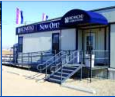
▲ Ramp with Step and Landing
